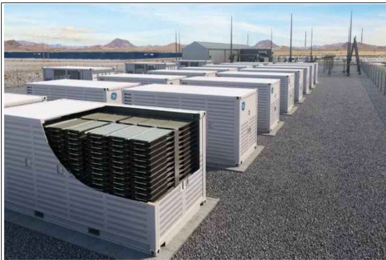
Figure 5: Typical BESS Arrangement
